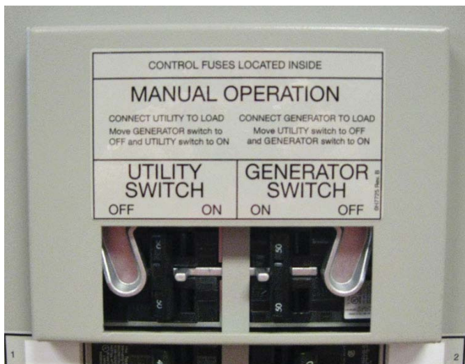
Figure 2 — Transfer Mechanism
