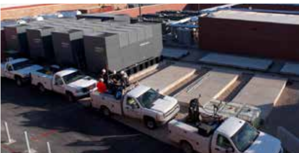
Pads poured for planned future expansion.
