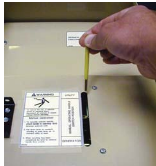
Figure 3.1 — Actuating Transfer Switch
